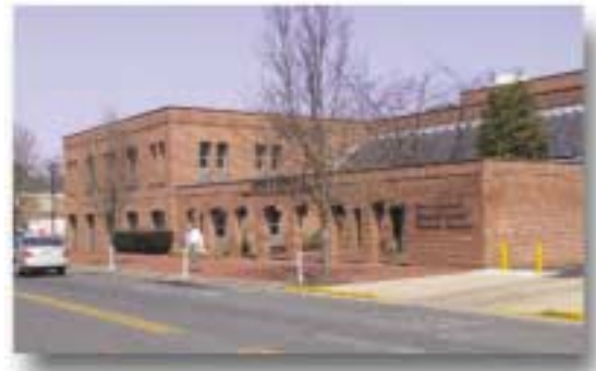
The District Court of Maryland, Centerville, is one of more than 118 government facilities affected by the performance contracts.
