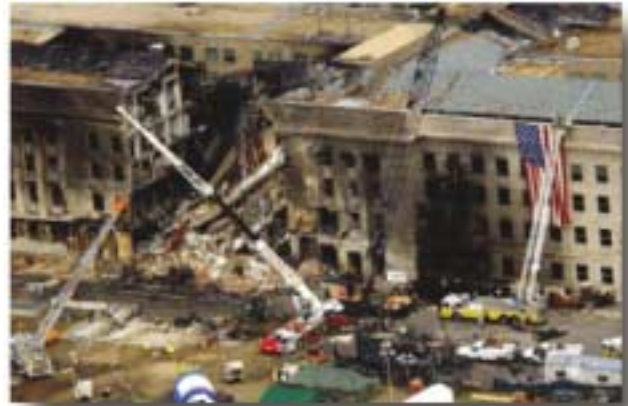
FBI Agents, firefighters, rescue workers and engineers work at the Pentagon crash site.
