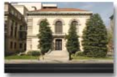
Hubbard Street building
