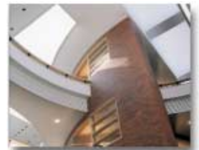
A daylighting program involves the use of light shelves placed on the west and south facades and a 10,000-square-foot atrium, which captures light through a skylight rising 12 feet above the roof line.
